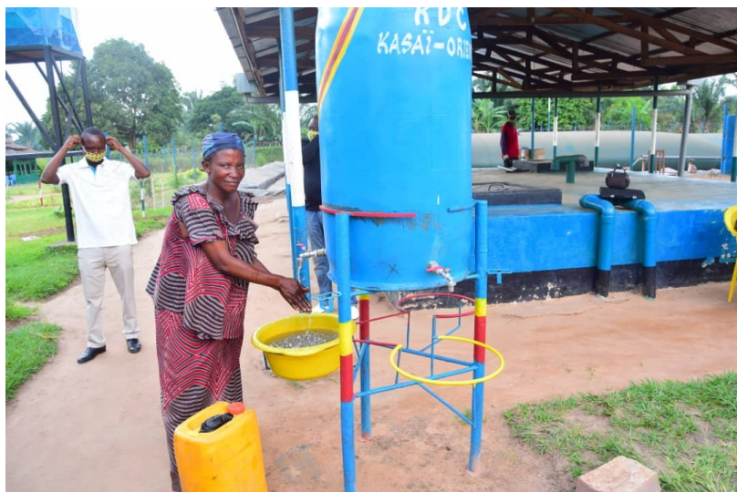
Installation de lave-mains publics
